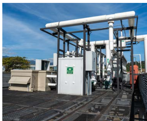
Photos 27 and 28: Example of chiller with R-290, in ROCHE Servicios S.A., Heredia., © GIZ/Gianfranco Vivi.
