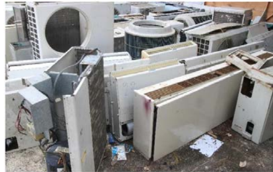
Photo 29: Obsolete refrigeration equipment, © GIZ
