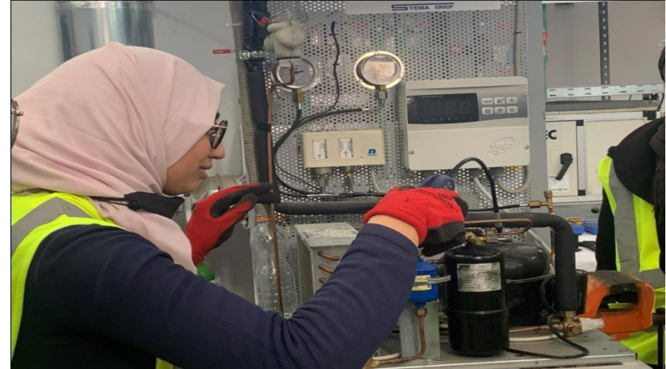
Electronic leak detection
