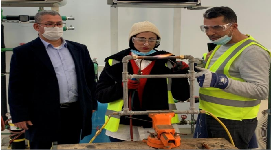
Brazing under nitrogen flow
